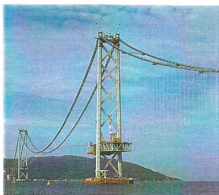
Nippon Steel has completed the main cable erection for the Akashi Kaikyo Bridge (center span: 1,990 m, the world's longest). The company developed 180 kgf/mm 2 high-strength steel wire and used some 50,000 tons of it for the two main cables.
